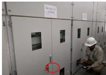
Fig. 6 PD location of 35kV 377 Switchgear
