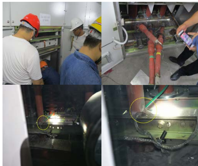
Fig. 7 B phase cable surface discharge traces of 35kV 377 Switchgear
